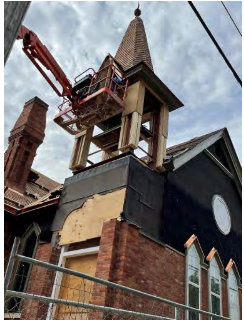
Hoisting the Belfry
